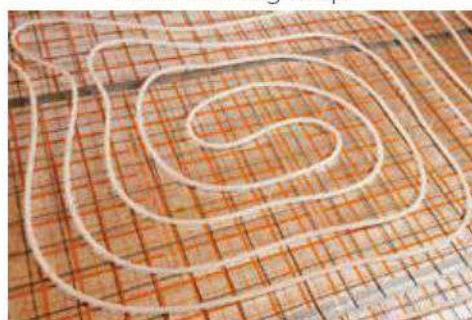
Floor heating loop
